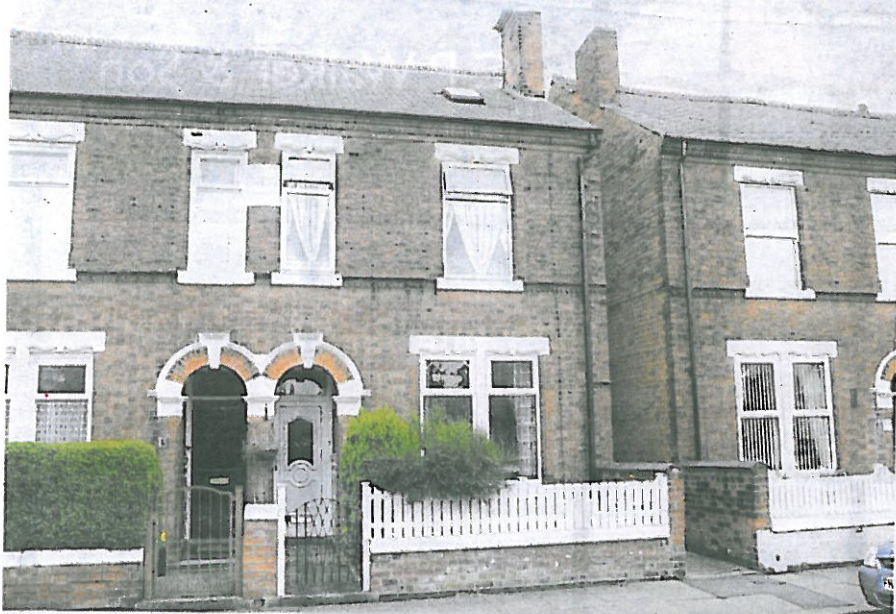
DECEPTIVELY LARGE: 17 Manchester Street, Long Eaton.
